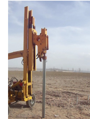
Steel post on-site testing
